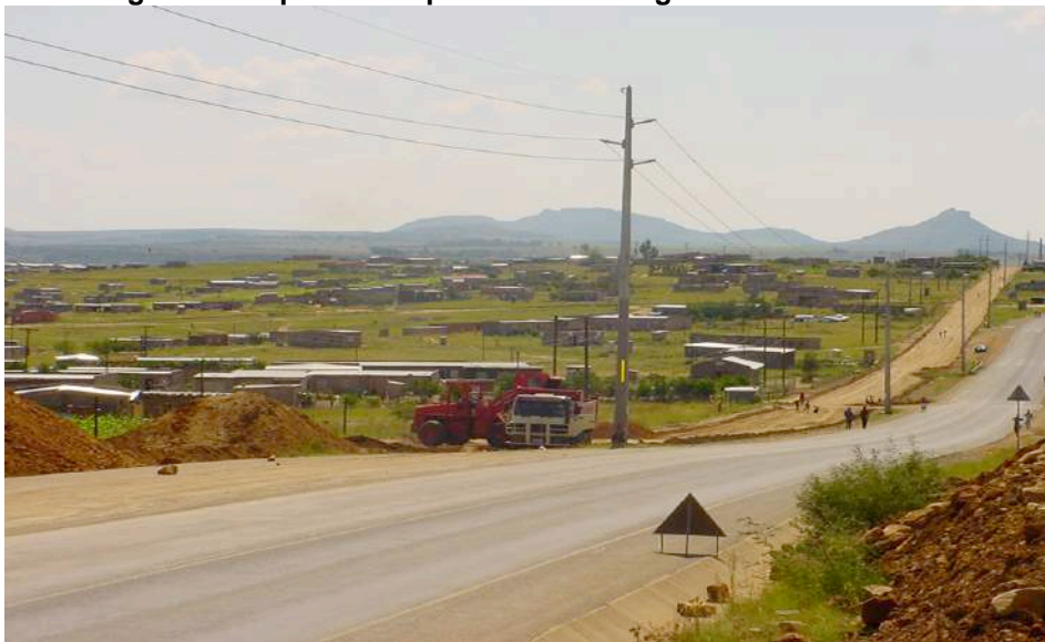
Figure 8: Rapid development on the edge of Millennium Park
